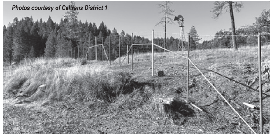
Caltrans' $8.8 million project along 2 miles of Highway 101 south of Willits is designed to guide wildlife toward the existing undercrossing at the South Willits Overhead Bridge, top right. Above left: The project also includes drainage improvements. Below: The 8-foot fencing has escape ramps for wildlife if they get trapped inside the fencing.
