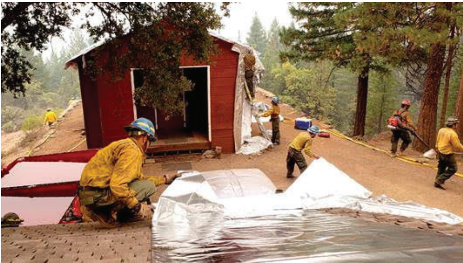
Above, left: Corpsmembers from Ukiah wrap the Post Creek Guard Station in foil to protect the 1934-built structures from the August Complex Fire. Above, right: CCC Ukiah Corpsmembers use hand tools to build containment lines around spreading flames on the northern edge of the August Complex fire. Below: A CCC Ukiah Corpsmember loads up with used fire hose before hiking the hose off the fire line.
