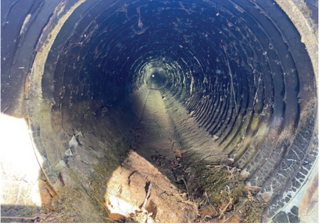
Above: Caltrans District 1 and other agencies assess damage caused by the Walker Fire south of Willits, on the freeway (left) and off (right). Below: Fire damage to a culvert and guardrail (at bottom) located on U.S. 101 south of Willits.
