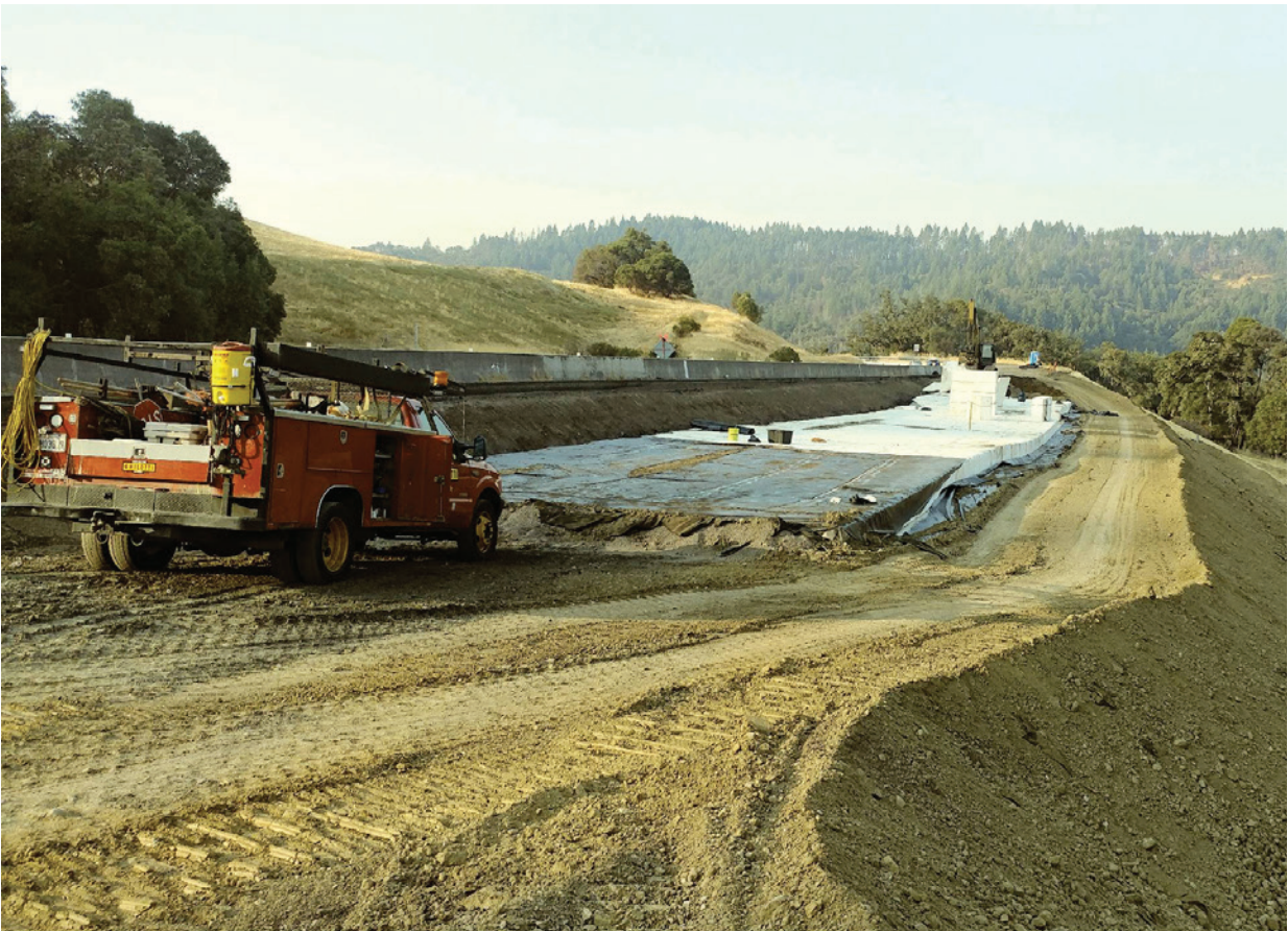
Above: Looking south over the area where the Ghilotti Construction Company has uncovered the light-weight fill blocks, and peeled back most of the membrane in preparation for the retaining wall. Below, left: Stockpiling dirt on the site to be used as back-fill. Below, right: A close-up photo of the 2-foot by 4-foot by 8-foot lightweight fill blocks that were once buried under the roadway.
