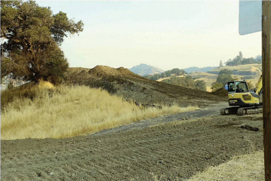
Above: Looking south over the area where the Ghilotti Construction Company has uncovered the light-weight fill blocks, and peeled back most of the membrane in preparation for the retaining wall. Below, left: Stockpiling dirt on the site to be used as back-fill. Below, right: A close-up photo of the 2-foot by 4-foot by 8-foot lightweight fill blocks that were once buried under the roadway.
