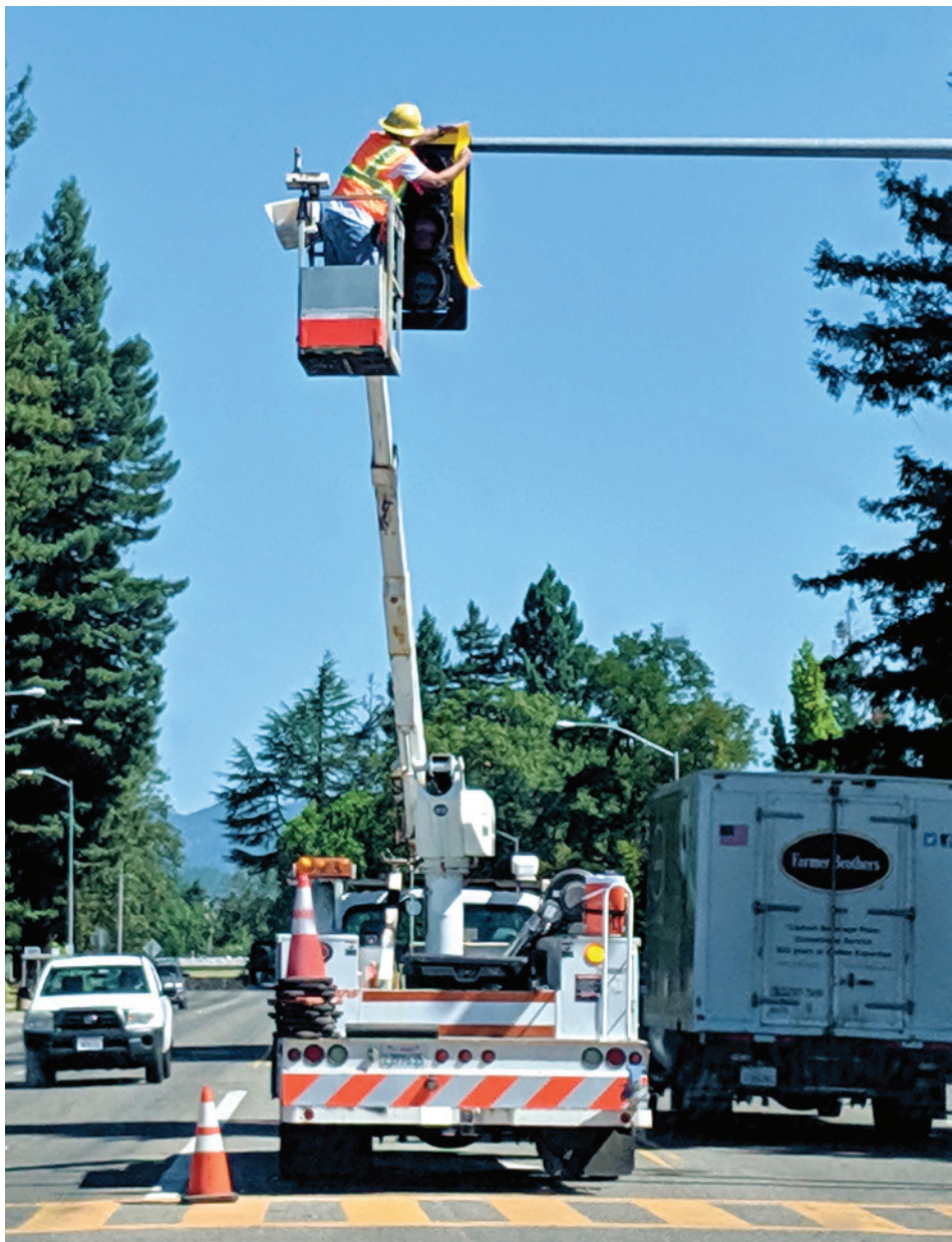
Above: Caltrans electrician Lance Miller, based out of the Ukiah maintenance yard, adds the new yellow reflective tape to the Burger King stoplight in Willits Monday.
