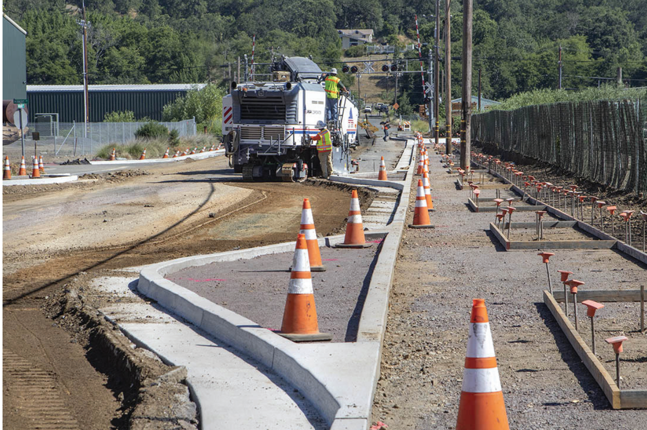
Above, from left: A worker on the road stripper helps guide the vehicle. In preparation, not only is the old pavement stripped, but so are several inches of dirt. The Chinese pistache trees will add color and much-needed shade to Blosser Lane. Below: These structures jutting out are designed to help slow the traffic near the school. Below, right: This road-stripping machine is making its first pass.
