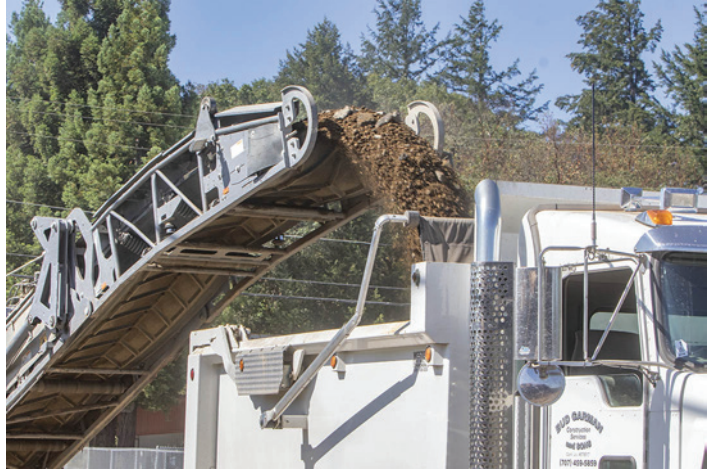
Above, from left: A worker on the road stripper helps guide the vehicle. In preparation, not only is the old pavement stripped, but so are several inches of dirt. The Chinese pistache trees will add color and much-needed shade to Blosser Lane. Below: These structures jutting out are designed to help slow the traffic near the school. Below, right: This road-stripping machine is making its first pass.
