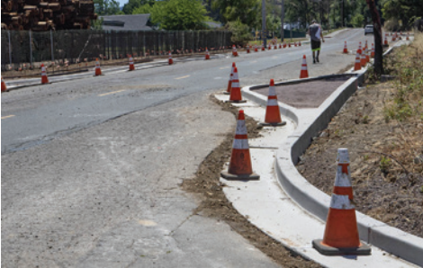
Above, left: Project Manager Jeremy Ronco of the Willits Public Works Department is supervising. Above, right: The sidewalks are also being redone to make them safer for the kids going to school. At left: Part of the roadwork includes new curbs, traffic "calming" projections, sidewalks, and irrigation for the trees that will be planted. Below: Bouthillier Construction, a local company, received the contract to repave the road.
