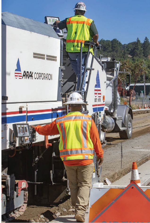
Above, from left: A worker on the road stripper helps guide the vehicle. In preparation, not only is the old pavement stripped, but so are several inches of dirt. The Chinese pistache trees will add color and much-needed shade to Blosser Lane. Below: These structures jutting out are designed to help slow the traffic near the school. Below, right: This road-stripping machine is making its first pass.
