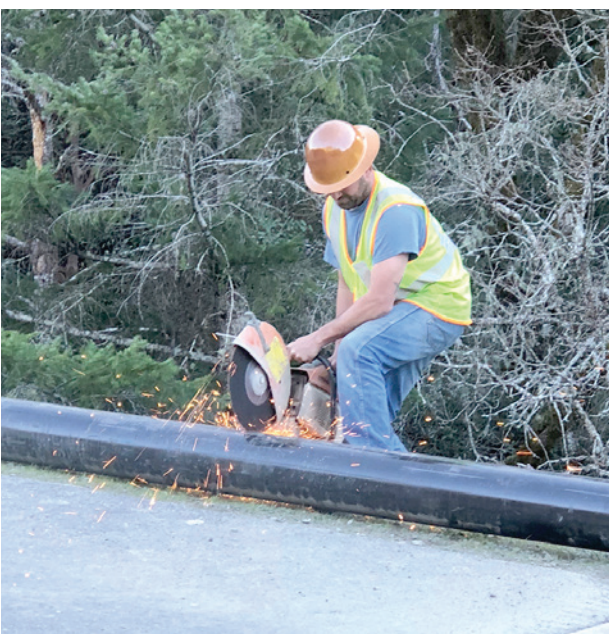
At left: Jeremy Sneed cuts a metal culvert to the correct length for the new culvert the crew installed out on Highway 128.
