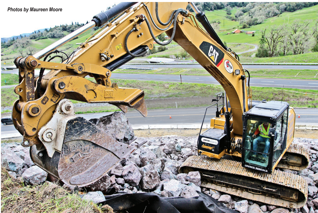
Above, from left: Argonaut Constructors workers pull filter fabric up the slope to cover the dirt, helping prevent sediment from getting into the watershed when it rains. Argonaut Constructors excavator operator Brian Torri on one of the excavators that is shuttling and placing rocks on the slope. Using excavators makes moving the giant rocks a manageable task. Below: Excavator operator Tim Noble swings the excavator arm, full of huge rocks, up the hill.
