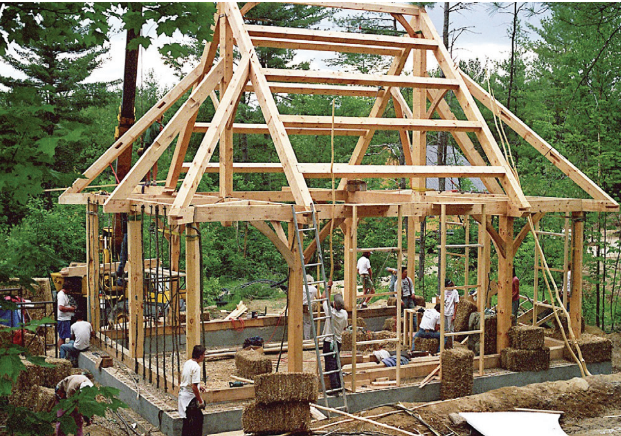
At top, left: Builders use straw bales as infill to a wooden frame that will be covered with earthen plaster to make a fireproof structure. At top, right: "Teamwork makes dreamwork," as a crew puts up heavy timber framing. Above, right: Proper use of earth in natural buildings can make them fireproof. Above: This home in the woods was built with Steve Chappelle's timber framing techniques.
