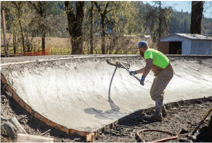
Above, left: Evergreen's project manager, Ben Hlavacek, smooths out the sides of the track that runs around the skate park. Above, right: The crew from Evergreen Skateparks lays forms and smooths cement for the new Laytonville Skate Park; the center is an enclosed bowl with the track, in varying elevations, running around the outside. At right: Roland and Jayma Spence stand in the track for the new skate park. Below: The framework for a curved bowl in the center of the park is nearly ready to be poured with concrete – Evergreen Skateparks' project manager Ben Hlavacek, comments: "For a park this size we usually wouldn't have a standalone enclosed bowl. So that's a different design aspect for us on this project. It turned out really unique and it'll be a lot of fun." At bottom: If the mound of dirt, people working, and wooden forms aren't clue enough, the "Evergreen Skateparks" sign lets you know you're at the Laytonville Skate Park on Harwood Road. Below, right: Roland Spence models the Laytonville Skate Park T-shirt, which is for sale on their website as a fundraiser.
