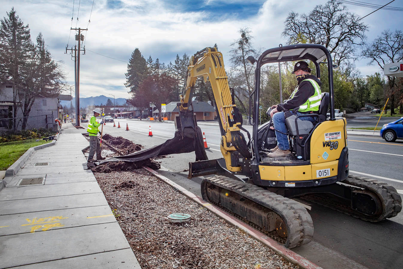
Above, left: The tree is in place and ready for the native soil to be refilled. Above, right: A small excavator rips up the material under the wood chips. At left: The pavers are carefully placed. Below: A landscape worker cleans out the area.
