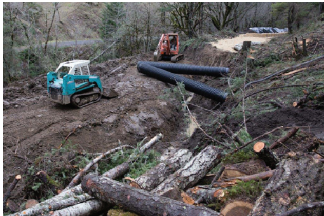
Above: Seth Coomer running the TL 26 and Stu Stewart in the orange Kubota prepare the ditch to install the culverts. Muir Mill Road is in the background. Below: Logs being yarded and hauled away by neighbor and volunteer, William Snipes, who also helped push mud around.
