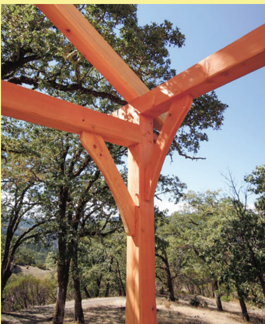
A detail of a new timber-framed building comprised of post and beams with graceful braces in the corners.
