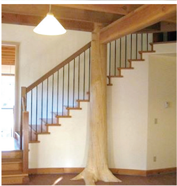
Above, from top: Sitting amongst the bones of a new timber frame is Dave Bixler, owner of Garfield Construction in Willits. Redwood beams crafted in Garfield Construction's shop on Highway 20 in Willits will be joined in the shop. A photo showing creative detail possibilities like utilizing an actual tree as a support post.
